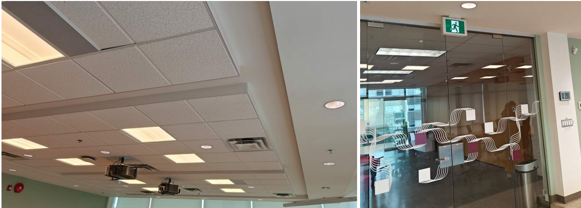
Figure 12: Existing Light Fixtures in Council Chamber 324
