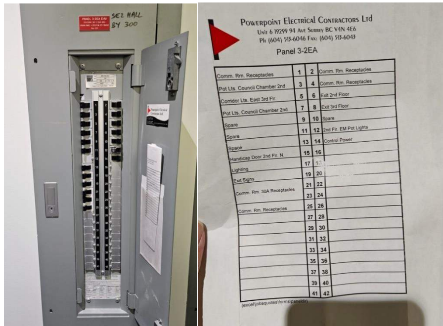
Figure 5: Existing Panel 3-2EA on Level 3
