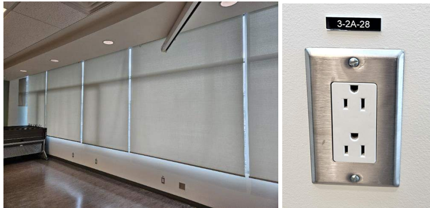
Figure 14: Interior Receptacles in Council Chamber 324 Sharing the Wall with the Patio Chamber
